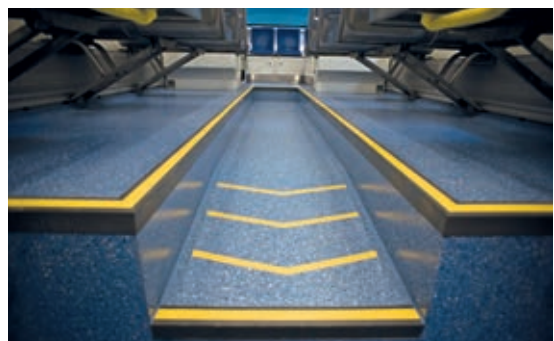
Stair nosing with signal stripes
