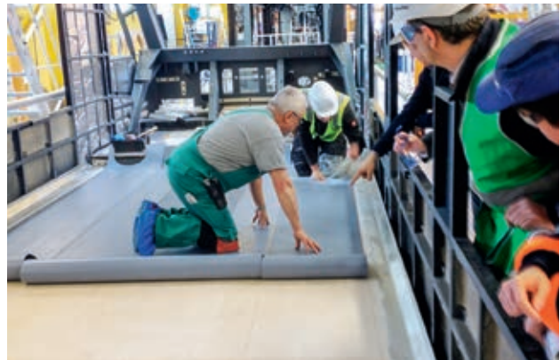
Ongoing nora nTx installation
